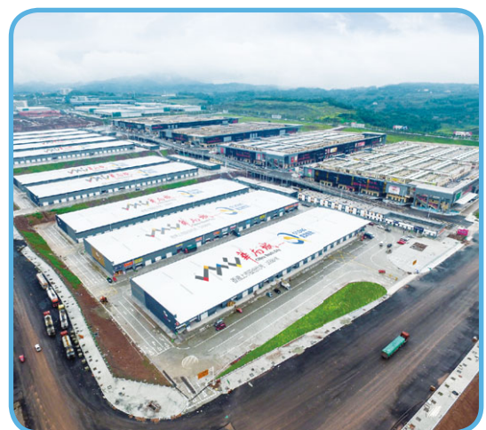
The logistics and warehousing services in CSC Chongqing 於重慶華南城的倉儲物流服務
